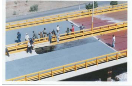
Laying the wear coat
