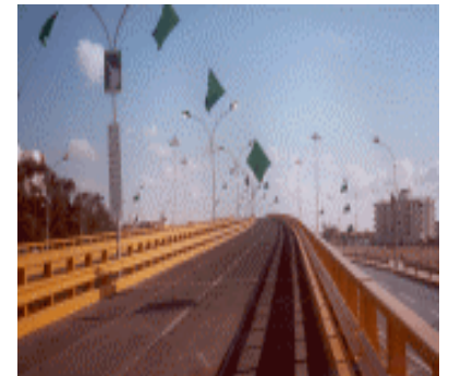
Roadway open to traffic in Benghazi, Tripoli road
