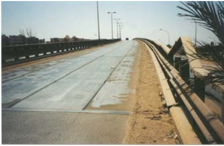
View of roadways as found
