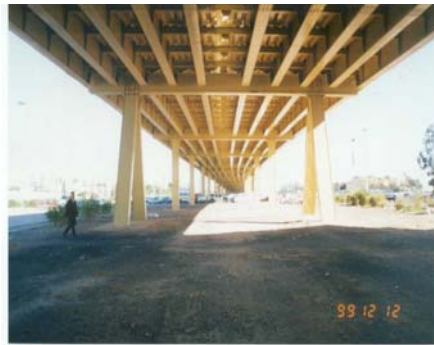
Bridge structure at handing over
