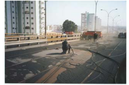
Roadways during surface preparation
