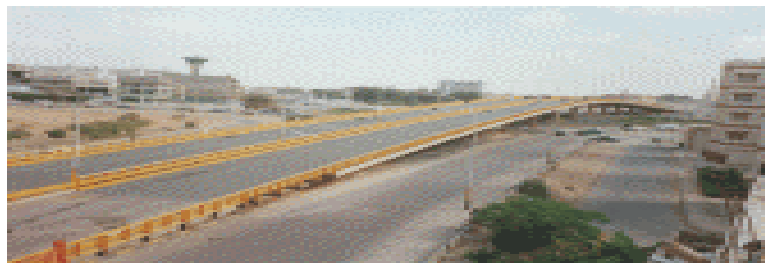
Roadway open to traffic in Benghazi airport road
