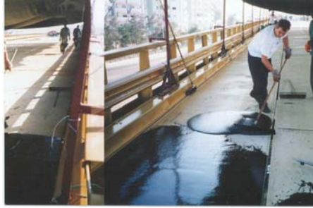
Laying the wear coat
