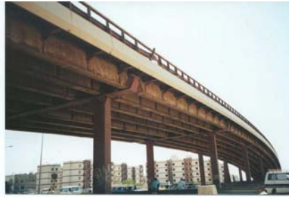
Typical steel structure as found
