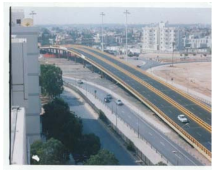
Roadway open to traffic in Tripoli airport road
