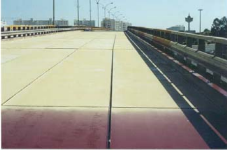
Roadway with priming coats
