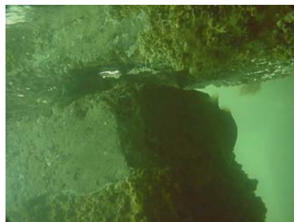
Typical ruptures between concrete piles and platform
