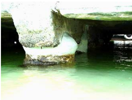
Typical ruptures between concrete piles and platform
