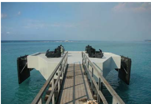
View of the Pier after rehabilitation
