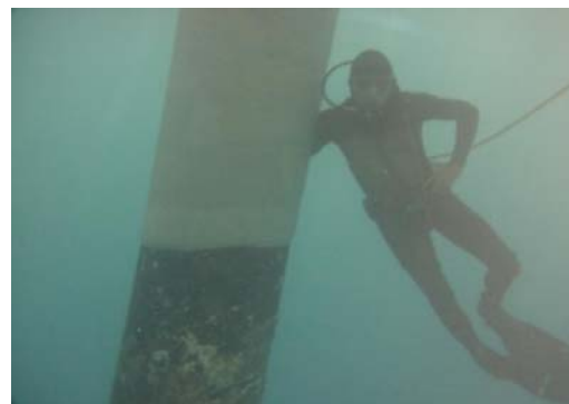
Subcom T.260 applied to one of the steel piles
