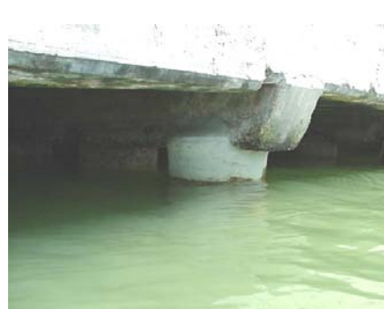
View of the rehabilitation with Subcom T.260 replacing concrete between piles and platform
