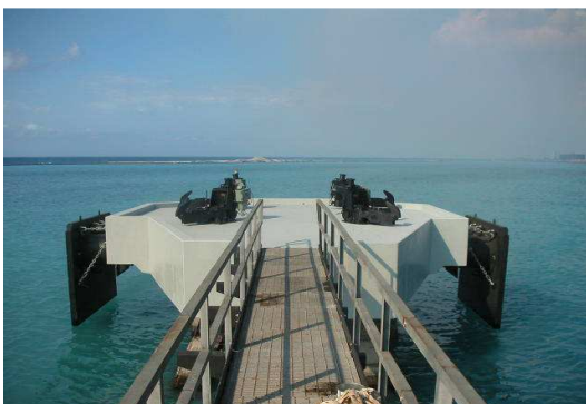
View of the Pier after rehabilitation
