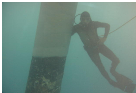
Subcom T.260 applied to one of the steel piles
