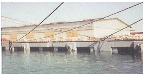
Coping beams repaired with #108 MORTAR and coated with #777 COAT.
