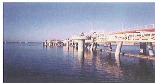
Splash-zone of petroleum pier coated with SUBCOM T.260.
