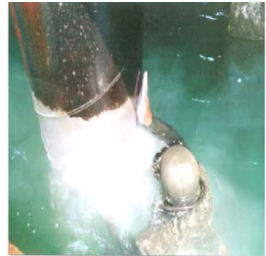
Application by manual spreading of SUBCOM T.260.
