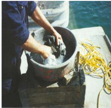
Hand mixing of the 2 components SUBCOM T.260.
