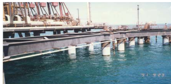
View of some coated piles.
