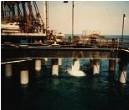
Underwater and splash zone grit-blasting.
