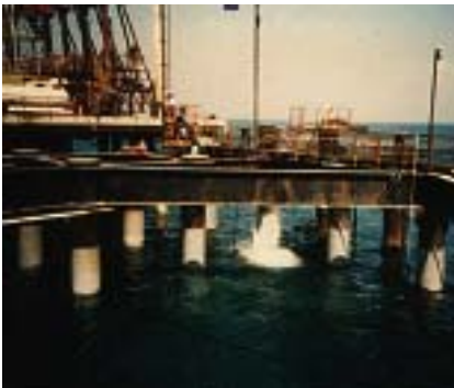
Underwater and splash zone grit-blasting.
