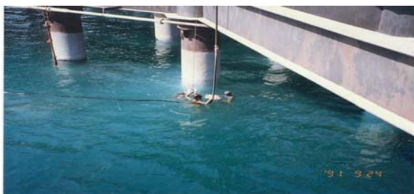
Application by manual spreading of SUBCOM T.260.
