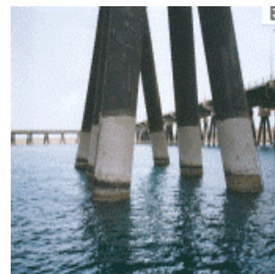
General view of the Jetty
