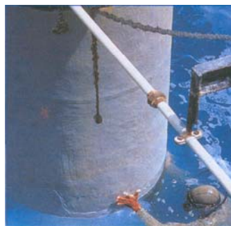
Spreading of SUBCOM T.260 on steel piles
