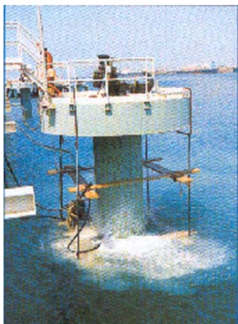
Grit blasting of splash zone
