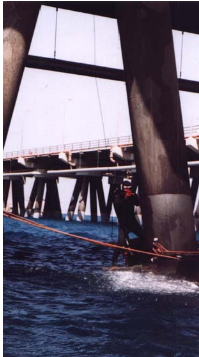
Grit blasting of splash zone
