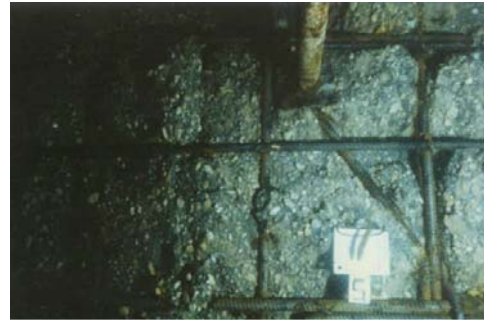
Underwater exposed reinforcement after grit blasting
