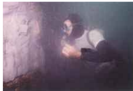
Spreading of SUBCOM T.260 on exposed reinforcement and concrete
