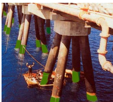
Spreading of SUBCOM T.260 on steel piles
