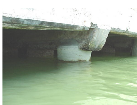
View of the rehabilitation with Subcom T.260 replacing concrete between piles and platform
