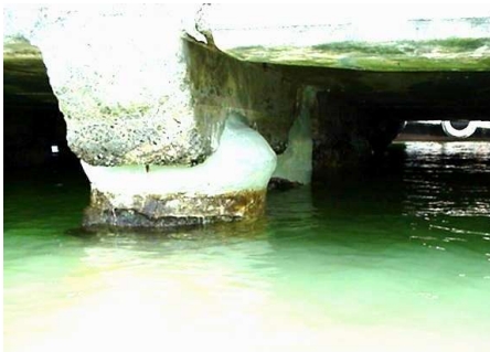
Typical ruptures between concrete piles and platform
