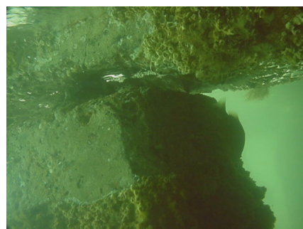
Typical ruptures between concrete piles and platform
