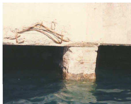
Coping beam heavily damaged with exposed re-bars.
